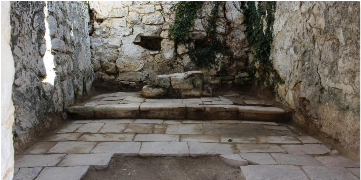
Image 2. Floor paved with stone slabs, remains of the altar in the presbytery
